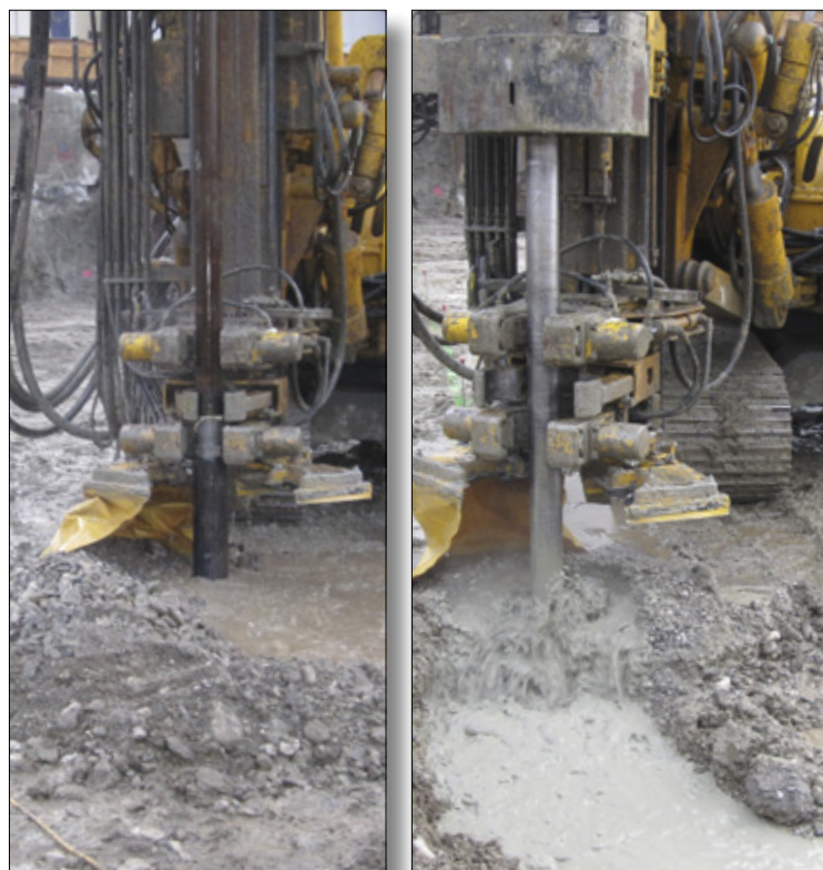
Drilling and jet grouting with Wassara Jet grouting hammer
