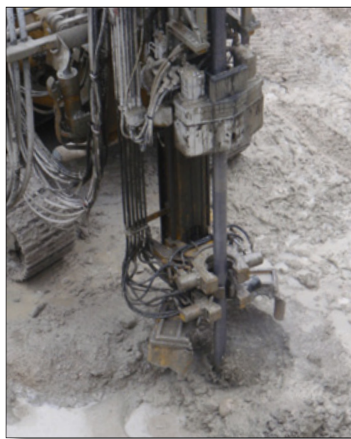
Jet grouting in soft soil
