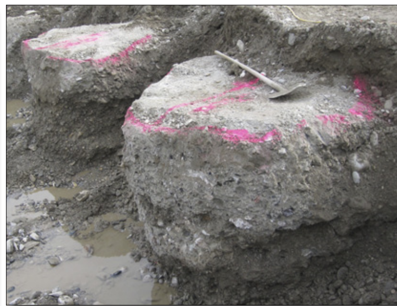
The result: Jet grouted cement columns
